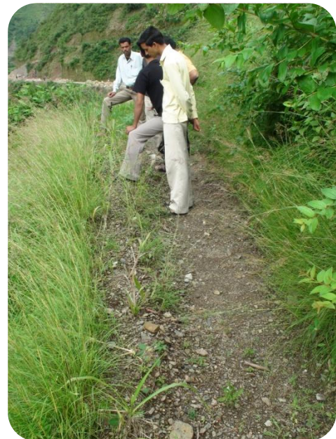
Recharge Structure: Contour Trench with slope adjustment of farm.
