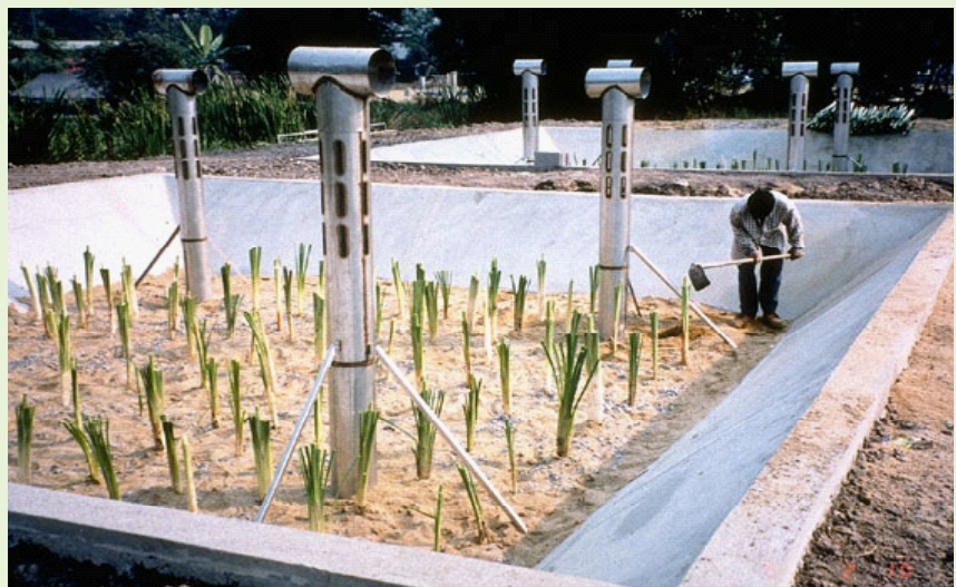
Photo 9: New installation of a constructed wetland with ventilation pipes at the Asian Institute of Technology (AIT) in Bangkok, Thailand. (Sandec, 1997)
