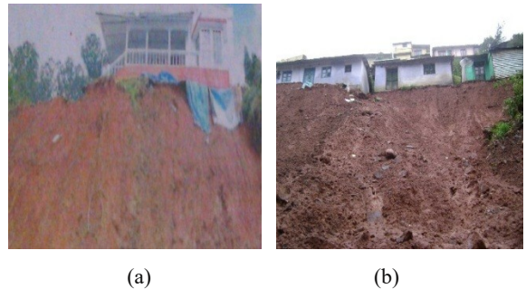
Figure 5. View of slope failure due to loading the slope at crest; (a) Kothagiri (b) Nondimedu
