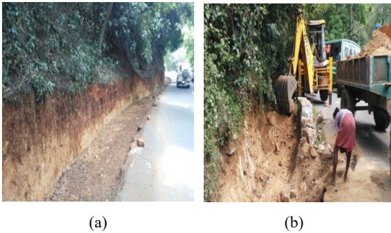
Figure 3. View of excavation of slope at toe; (a) & (b) along Mettupalayam - Coonoor road network
