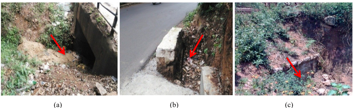
Figure 6. View of blocking of surface drainage pipe and drainage culvert ; (a) & (b) along Mettupalayam–Coonoor road network (c) Aravankadu location
