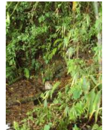
Fractures in rock near the spring
