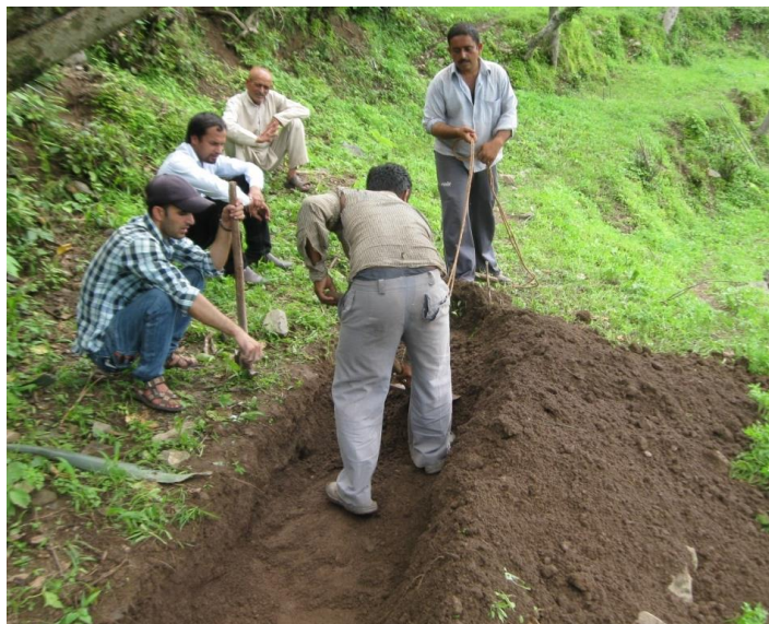
Figure 10: Staggered trenching on the slopes (Source: PSI, Dehradun)
