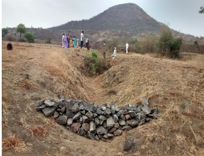
Figure 9: Stone bund structure constructed in a stream channel (Source: Velu GP, Maharashtra)
