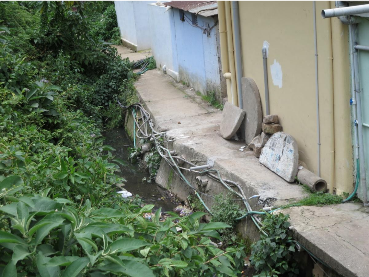
Figure 13: Sewage being drained into the stream
