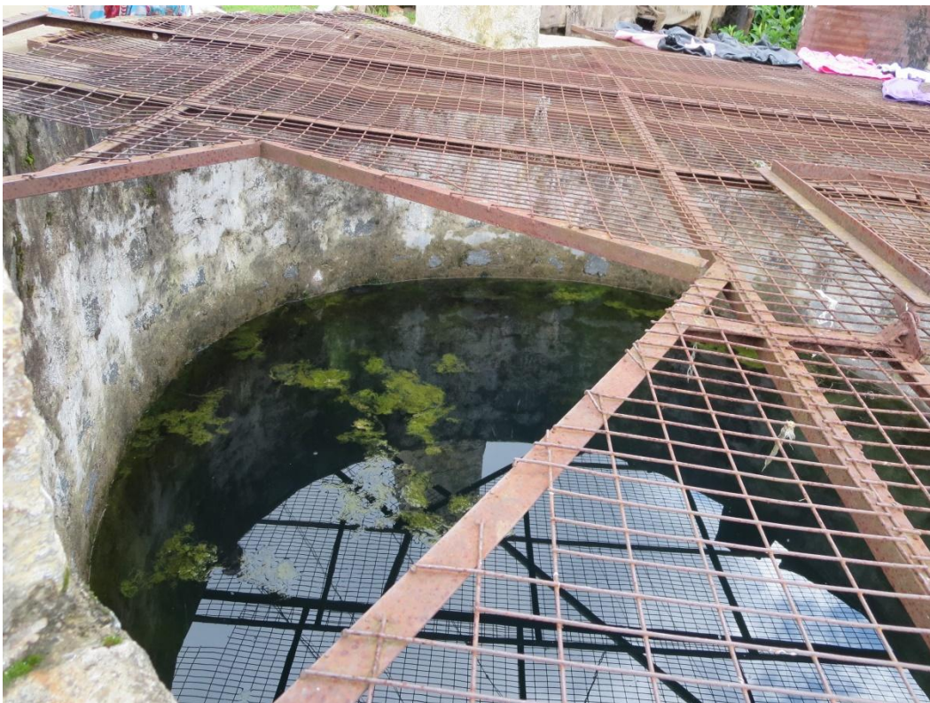
Figure 11: The community well used by the residents of Indira Nagar
