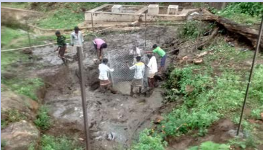
Construction of spring box
