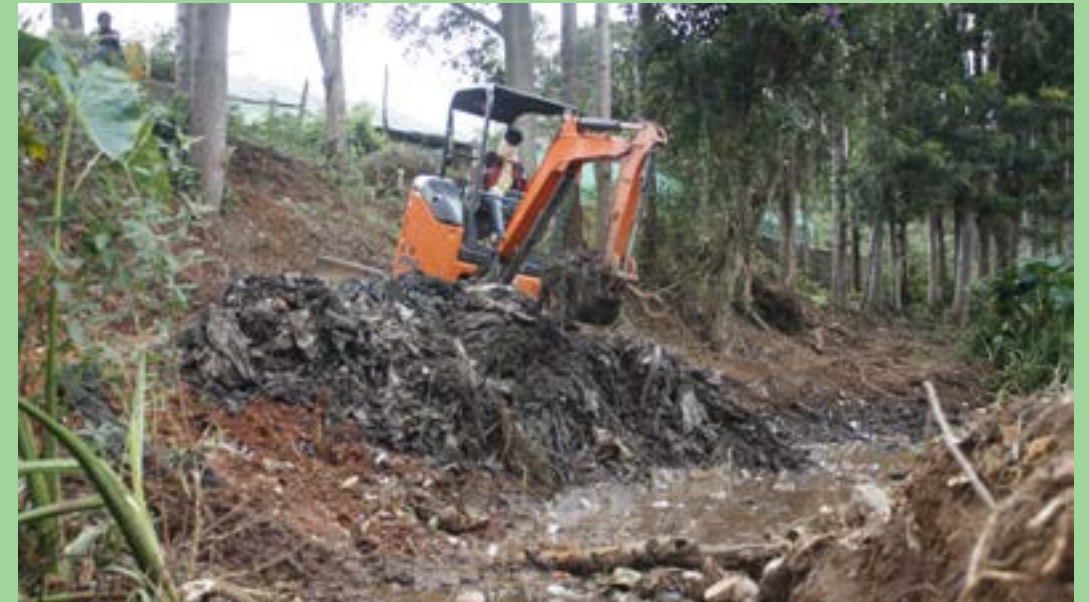
Earth moving machine in operation
