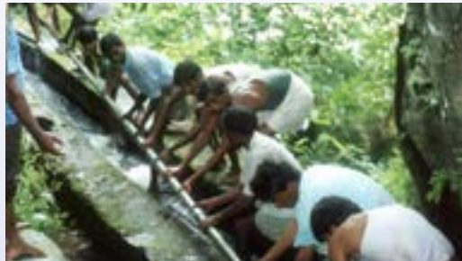
Laying the pipeline at Kilcoupe
