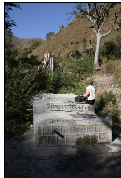
Structure to store and measure spring discharge
