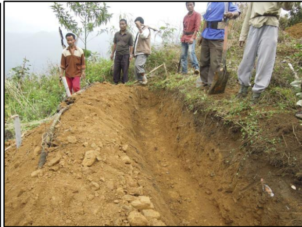
A trench being dug in a recharge area at Okthem
