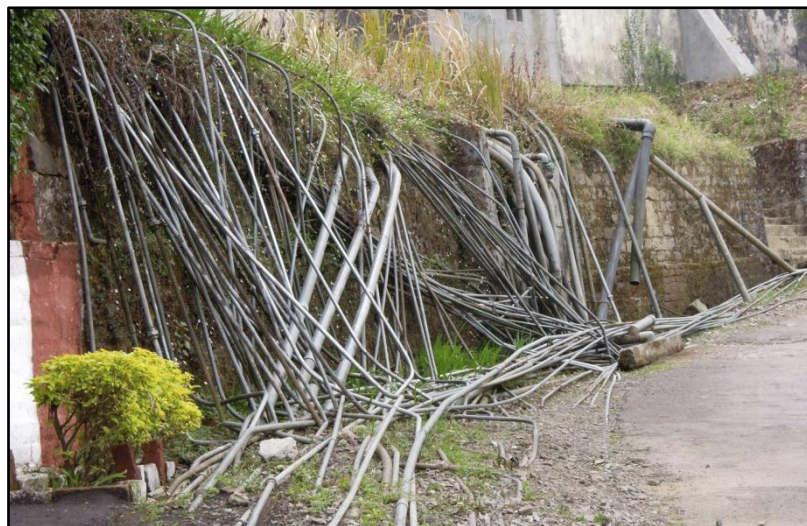
A typical chaotic setup of pipelines used for distributing water tapped from springs in the hills, Mokokchung, Nagaland
