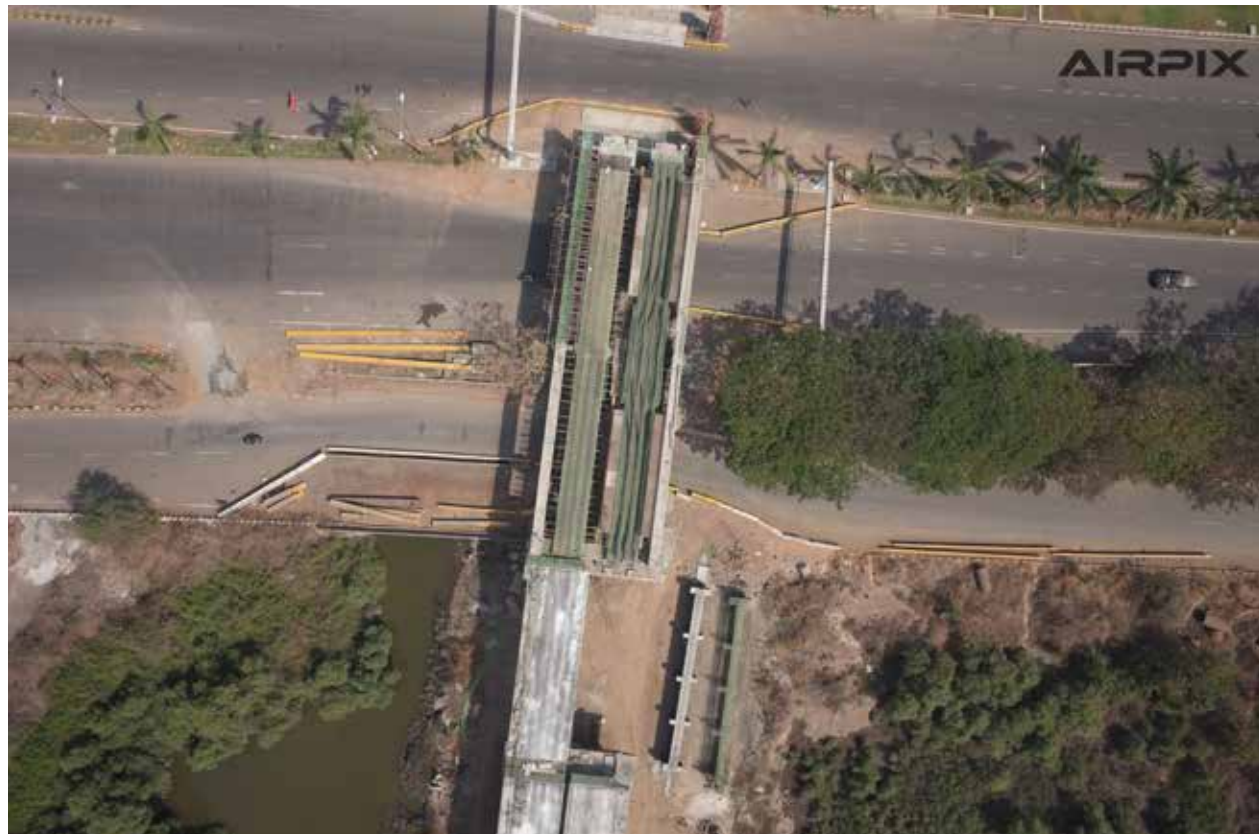
Figure 1: Existing status of a ROB along the Seawoods-Belapur-Uran project
