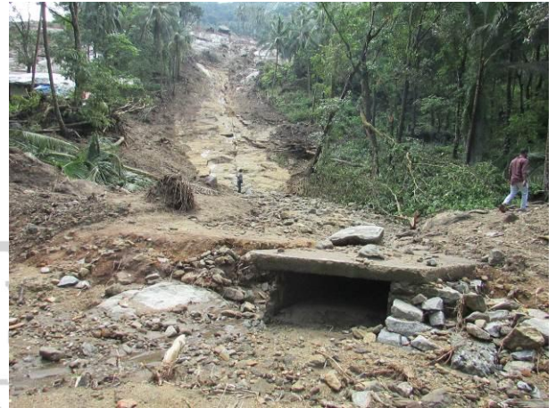
Fig. 12: Damaged road and culvert due to the debris flow
