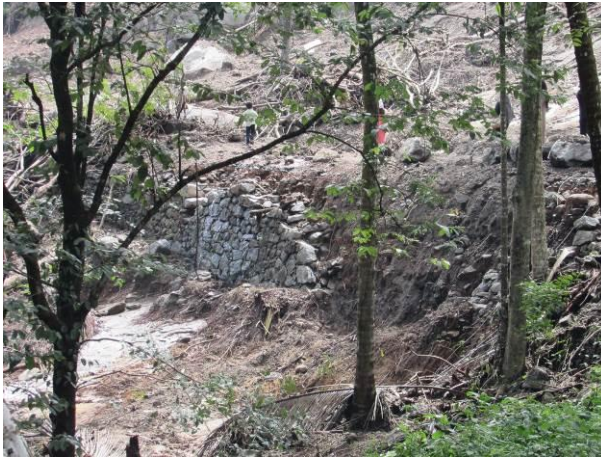
Fig. 11: Damaged RR masonry retaining wall of the road.
