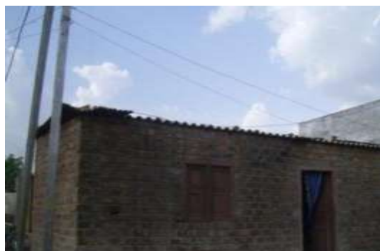
Cement Sheet as Roof Tops
