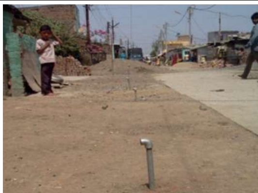
Water connection in front of each house (non-operational)
