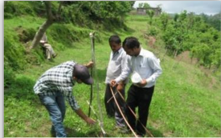
Laying out of Trenches
