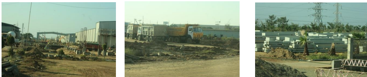
Fig 14. Construction activities within the core zone
