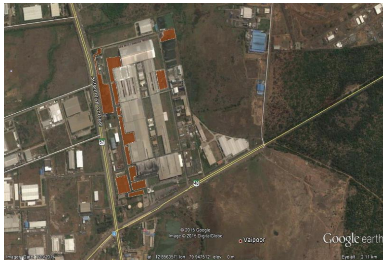
Fig.13. Construction/expansion activities indicated in 'red'
