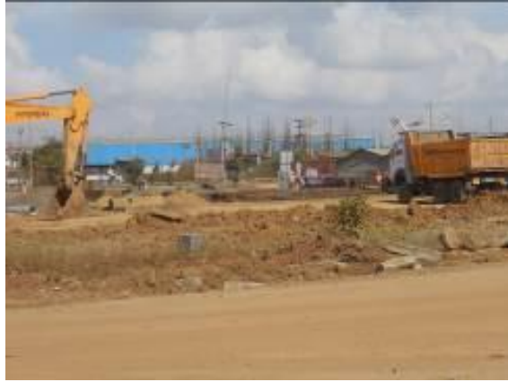
Fig 8. Construction activities at the core zone
