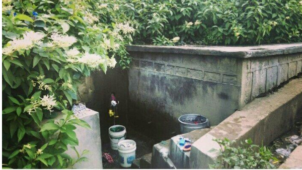
Spring-box right next to sewage at Baptist colony
