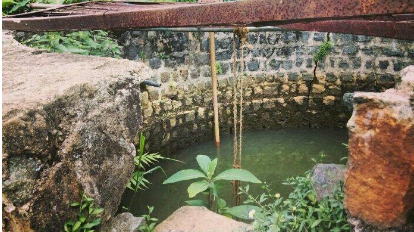
Panchayat well that supplies water to Govt. hospital, Kotagiri market, Darmona
