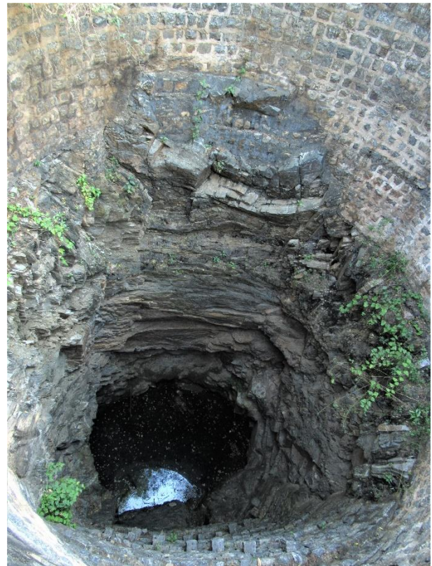
Photo 8: Old well exposing the subsurface geology in Poochamarathur village
